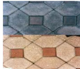
Paver Stone Restoration
